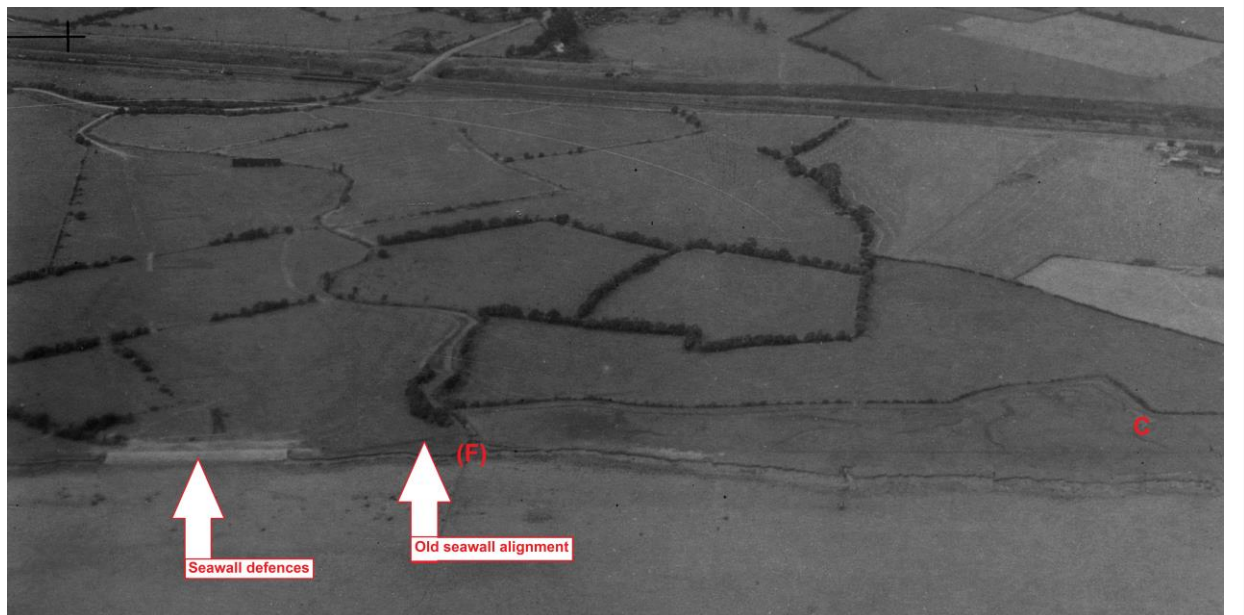
Photograph B: showing 1951 Seawall construction
